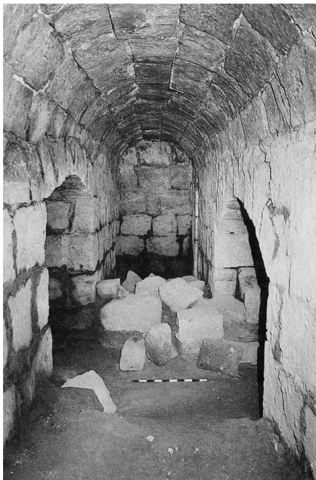
Fig. 5. Beth Shean / Scythopolis, subterranean vaults of the Roman temple attributed to Dionysos (after: Foerster - Tsafirir 1992: Fig. 12, top [p. 8]).
